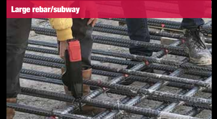
Multiple rebar tying
