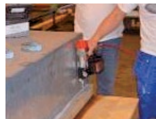
Light Steel Roof to Structural lumber
