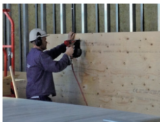
Plywood to Metal Stud
